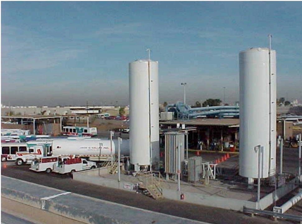
Station Shown has two 30,000 gallon Storage
